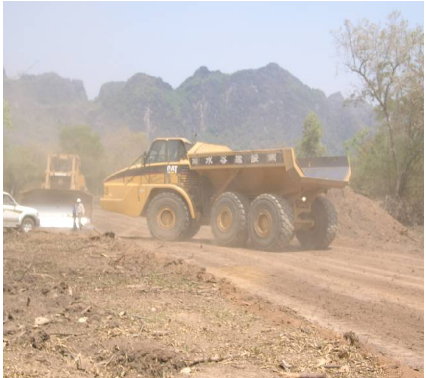
Figure 5. Construction site Downstream Channel (Nam Phit) (H.D.B)
